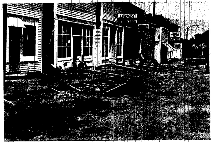
NEW SIDEWALKS went in on the west side of the main street in Hoskins the past week. Planks were used to enter business places while the concrete was hardening. This is one of the improvement projects for the centennial.
